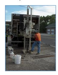
with a soil sampling device attached to it. At each sampling location, the sampling device was extended into the ground to collect soil samples to depths up to 20 feet. Each soil sample was reviewed by a geologist, who tracked the type of soil found (e.g., sand, clay, etc.), and the attributes of the sample (e.g., whether staining was noticeable, or the color of the sample, etc.). A total of 180 soil samples were collected from 49 borings.
