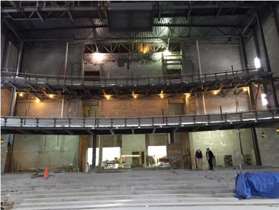
View from Stage prior to scaffold erection
