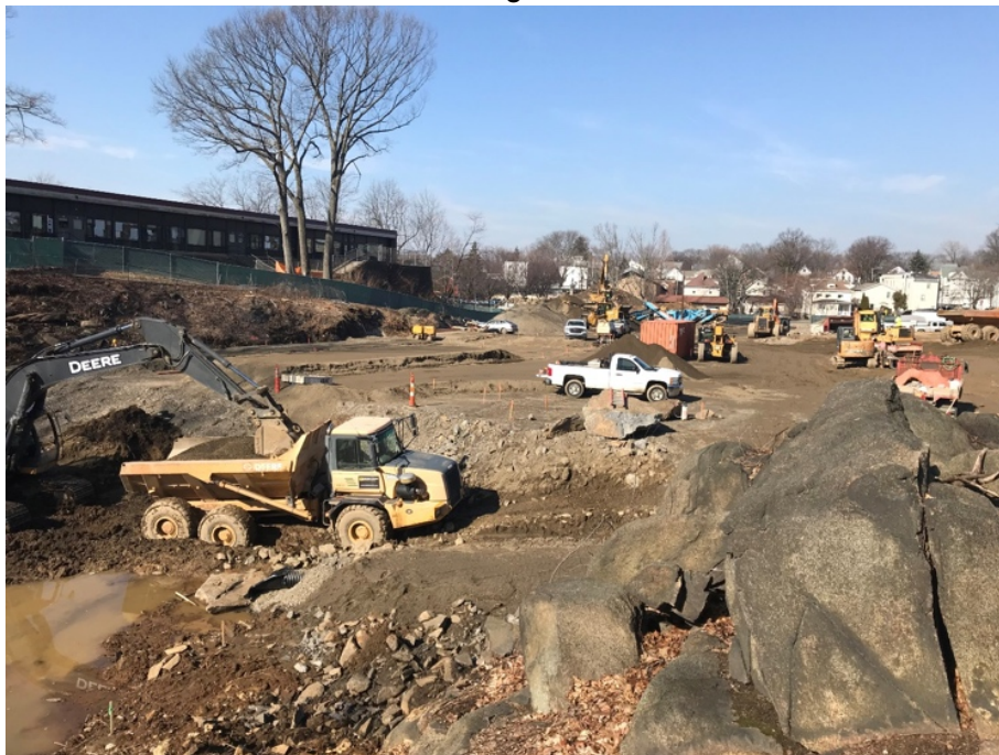
View of site looking East – 2/21/2018
